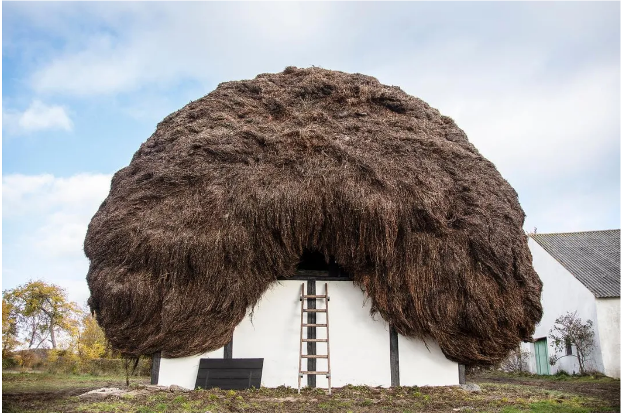
A single roof takes three people two months to complete. That's 90 tons of eelgrass spun into rope, wrapped around the top of each timber frame and piled on. Fotograf Kjetil Løite
